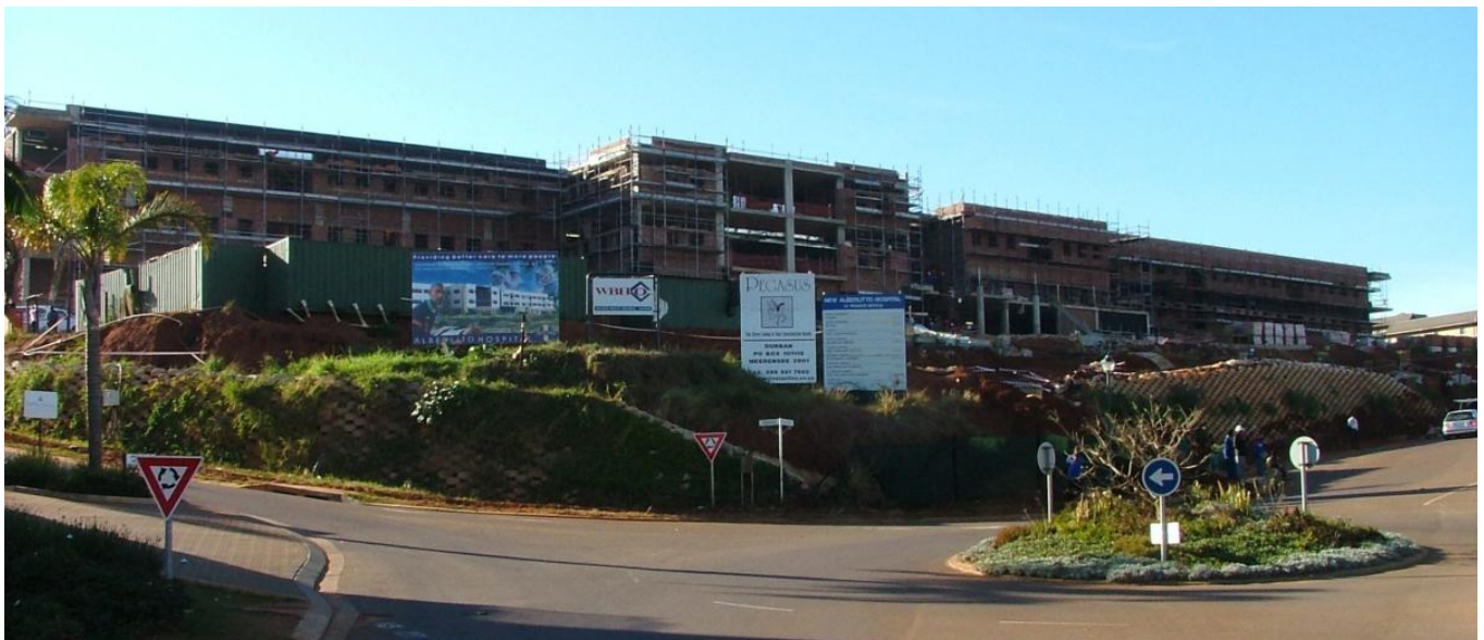
ALBERLITO HOSPITAL | CONSTRUCTION PROJECT MANAGEMENT | 2005-2006
